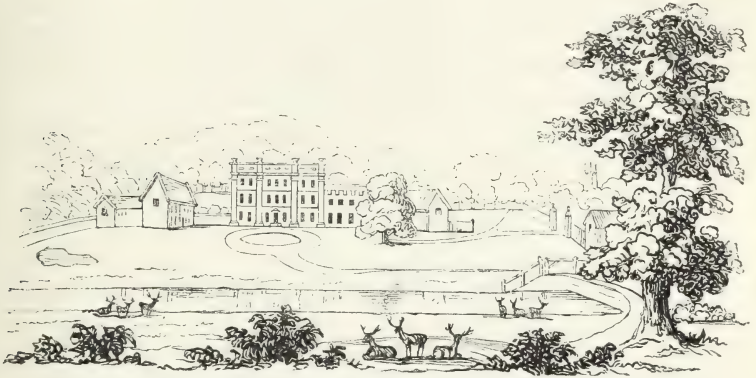
[Fig. 166. View of the house at Harlestone Park, previously to Mr. Repton's improvements.]
